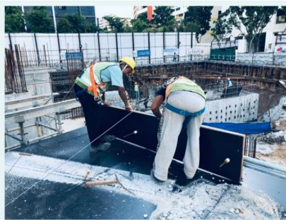
Workers using SRL when working near unprotected edge.
