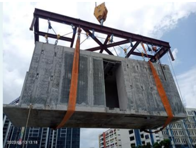
Securing webbing sling around the PPVC for additional measures.
